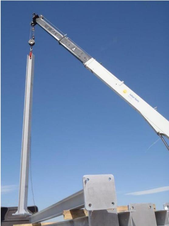
*On/off-track crane for installation*
