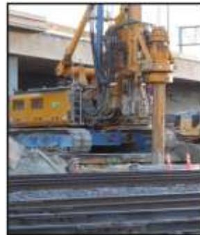
Right: Drilltech off-track OCS Drill Rig
