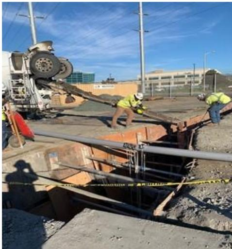
TRC placing encasement for Circuit #1 at EGS
