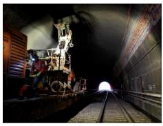
Tunnel 4: OCS Anchor Bolt Installation using Template (left) and Exposed Brick from Notching (right top)
