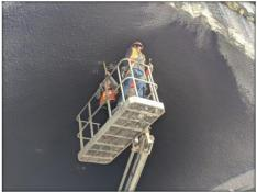
Tunnel 2: OCS Anchor Bolt Testing
