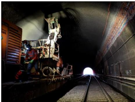
Tunnel 4: OCS Anchor Bolt Installation using Template (left) and Exposed Brick from Notching (right top)
