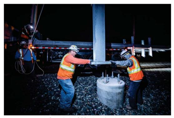
Crew placing OCS pole on foundation
