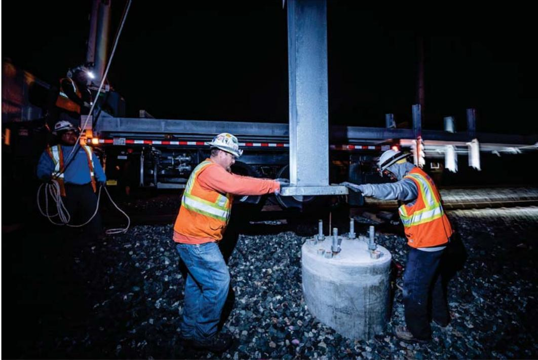
Crew placing OCS pole on foundation
