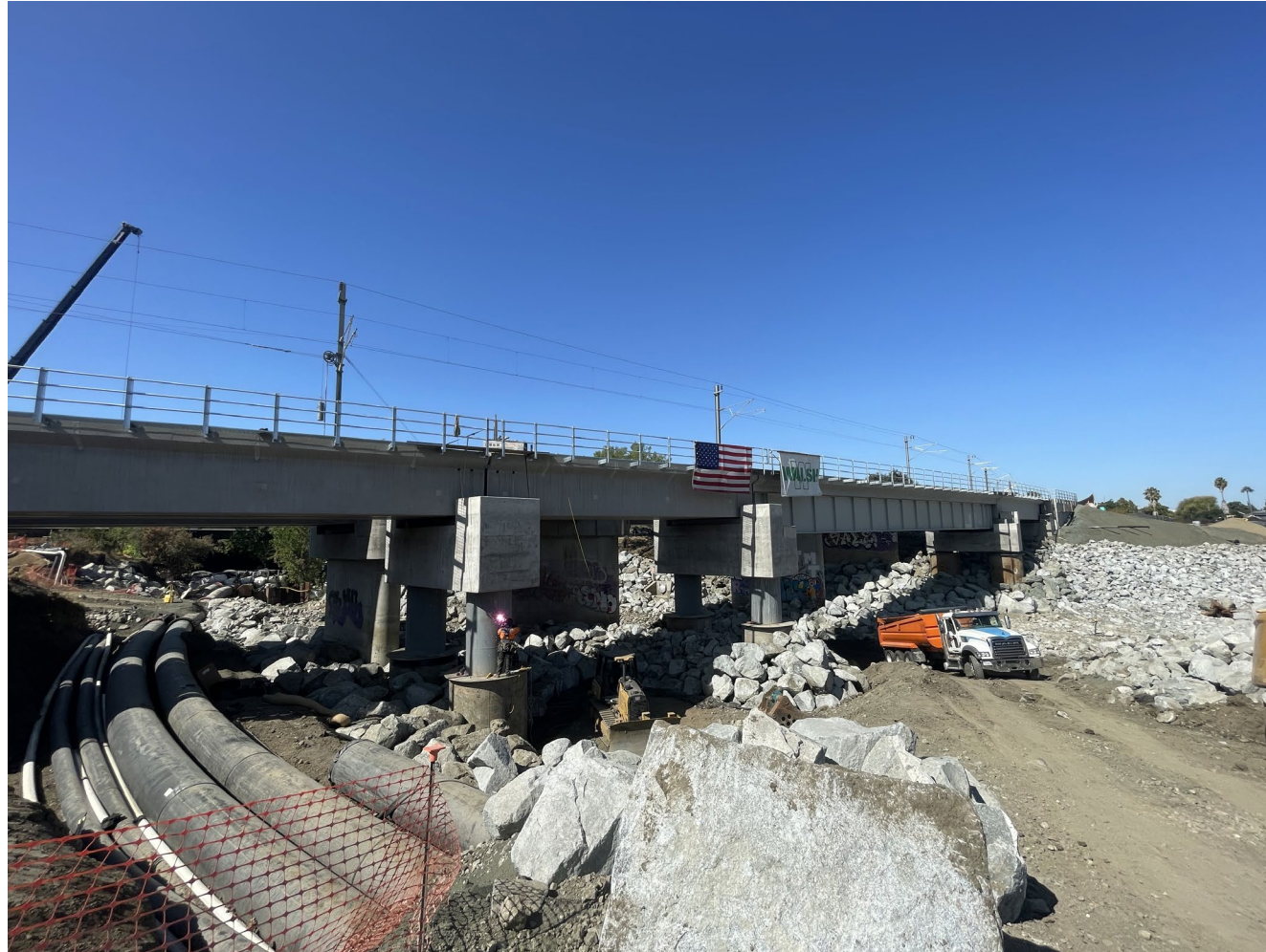
Complete MT1 Bridge Structure and Deck
