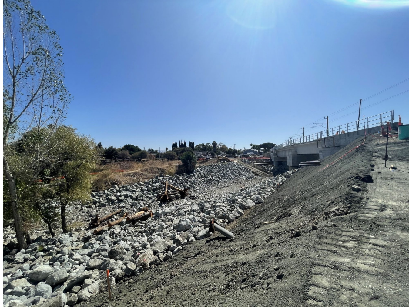
Stream Restoration and HMMP Installation
