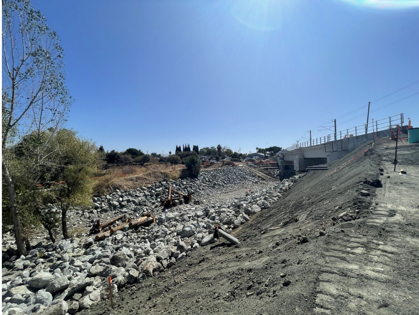
Stream Restoration and HMMP Installation
