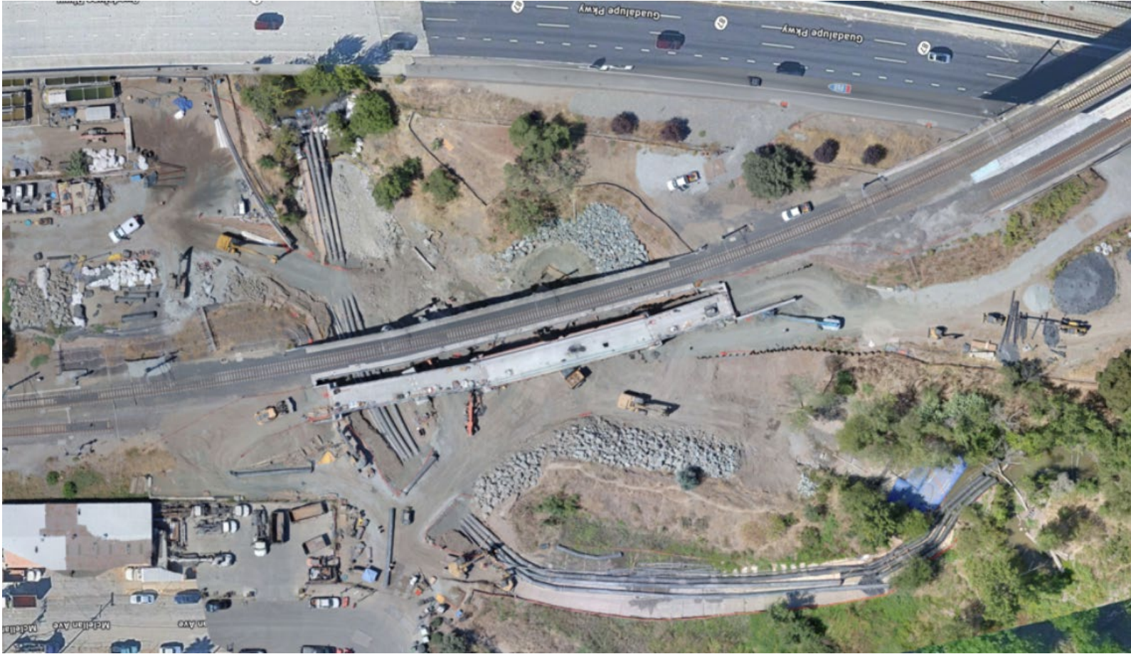
Project Overhead Photo – Summer 2026
