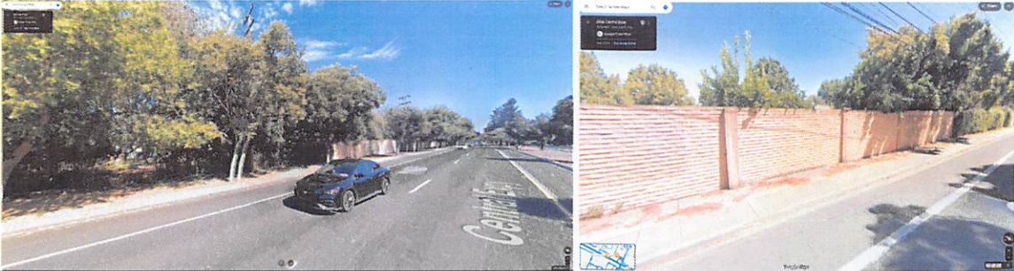
Attachment B. Existing standard wall in adjacent neighborhood
