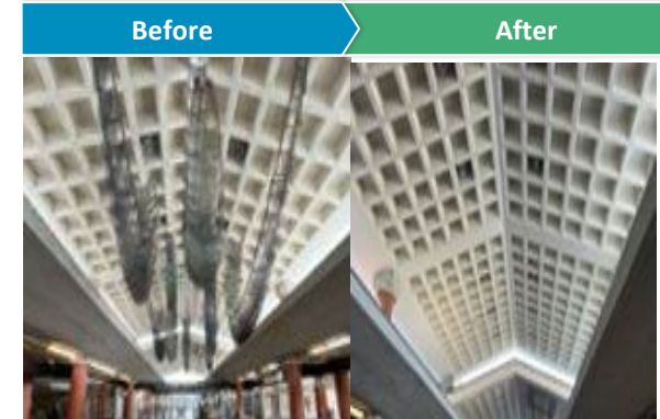
Removed artwork from concourse ceiling
