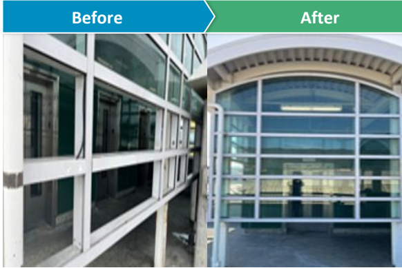
Installed glass window at 3rd floor, garage
