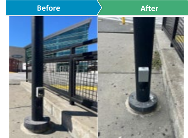
Repaired vandalized junction box at base of pole
