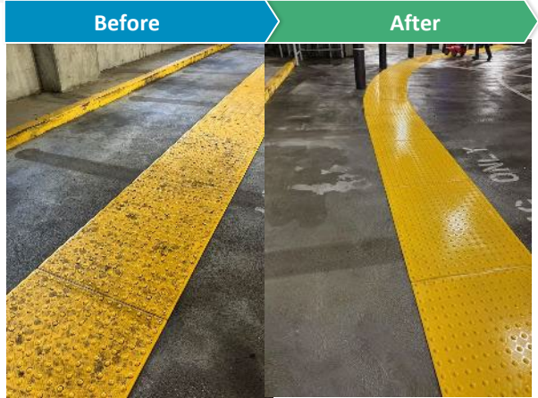
Pressure washed truncated domes at garage
