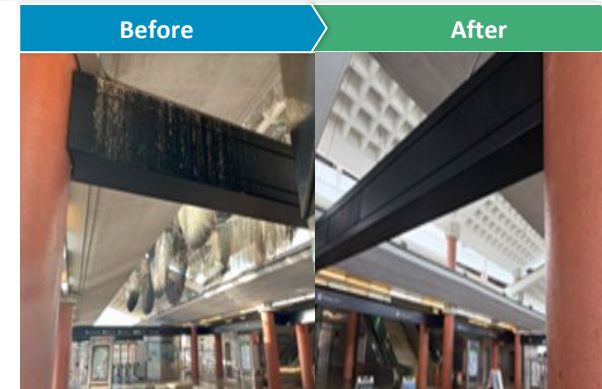
Cleaned away pigeon dropping from beams at concourse
