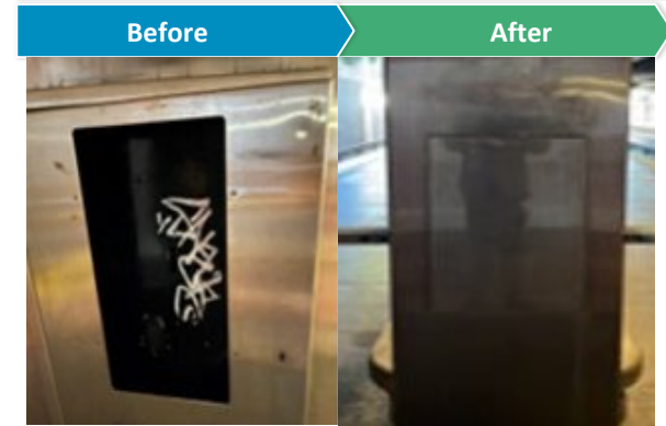
Installed new cover onto obsolete phone wiring cabinet to prevent littering
