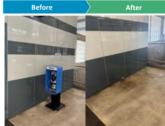
Removed obsolete phone booth
