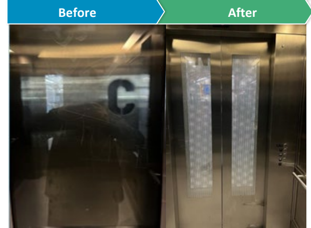
Replaced glass with screen doors to prevent vandalism
