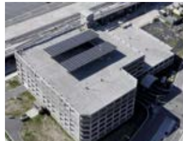
Energy Storage Solutions
