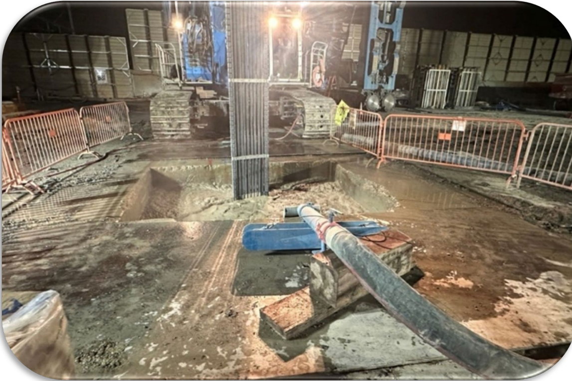
Milling Operations for Y-Panel
