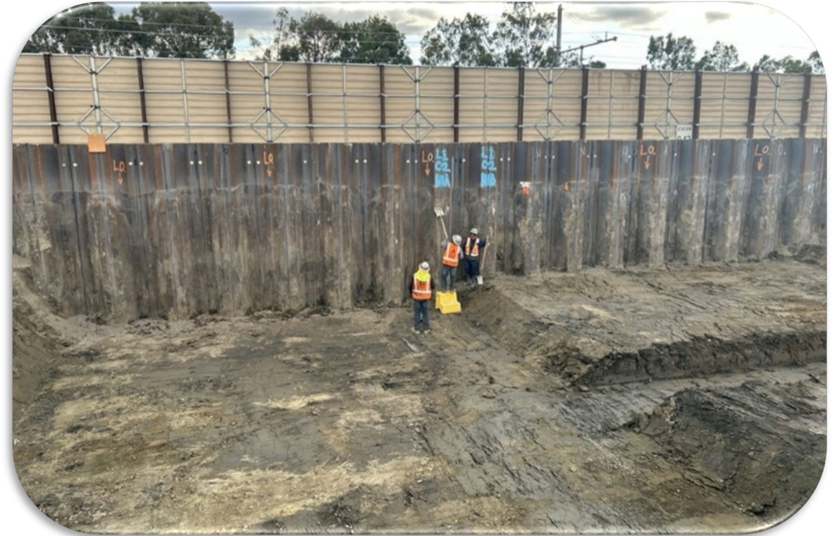
Mass Excavation Progress within Sheet Pile Area
