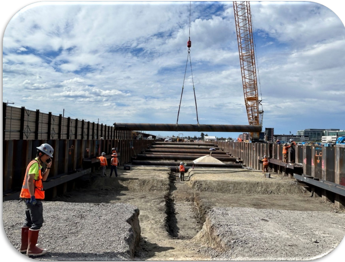
Installing Struts for Bracing on Sheet Pile Wall
