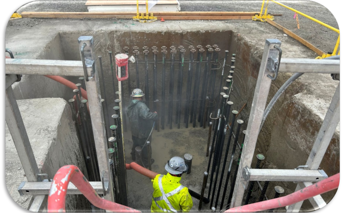
Pressure Washing of Y-Panel
