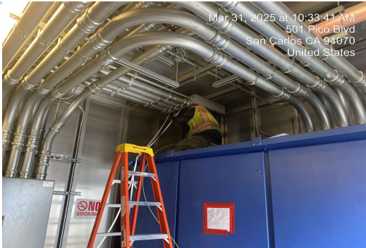
Anvil Power pulled mule-tape in-preparation for PG&E's power cutover.
