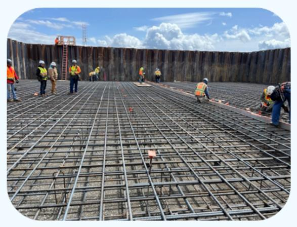
Placing reinforcement bars, or rebar, in the detention basin
