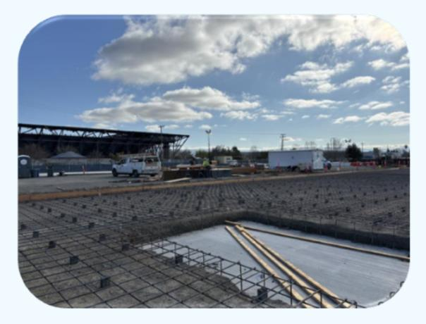
Constructing a desander slab which will hold equipment that separates materials not suitable for construction from excavated soil
