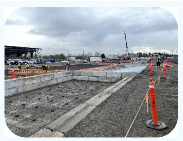
Poured concrete slabs for construction equipment
