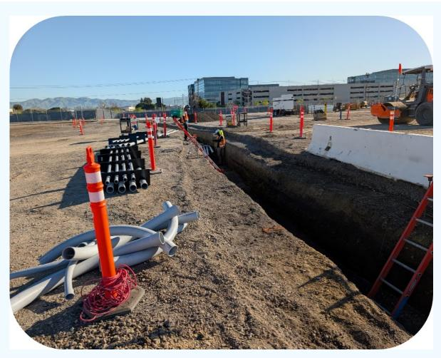
Trench and electrical conduit installation needed to provide electricity to various on-site facilities
