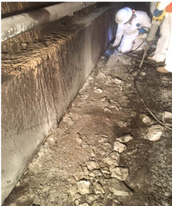
During the removal of shotcrete
