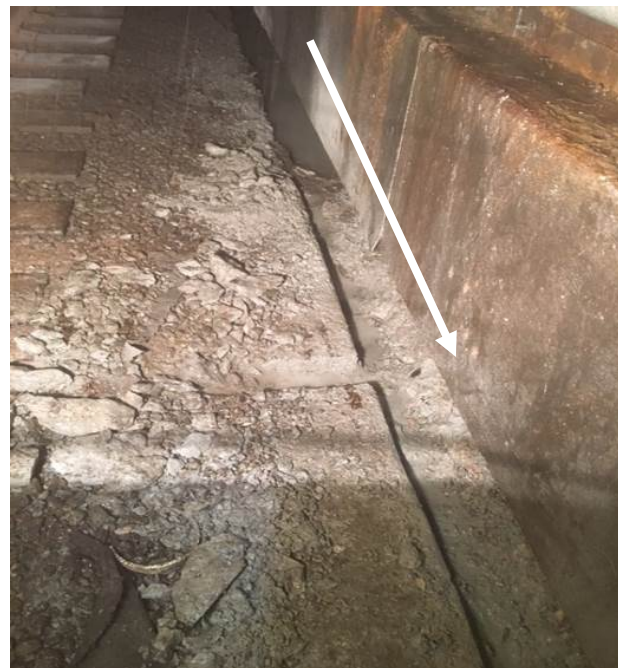
Trough restored to aid drainage
