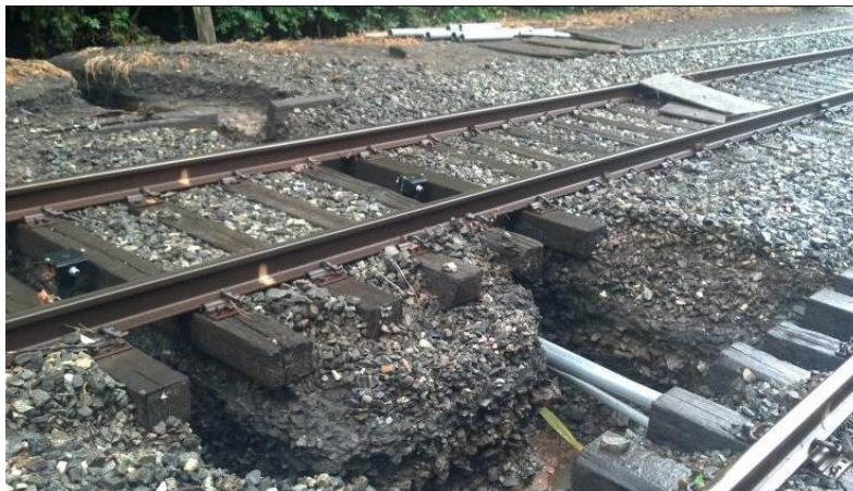
Trenching or Boring of a Signal Conduit
