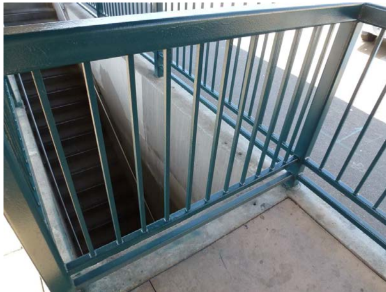
Hand railing along San Mateo platform
