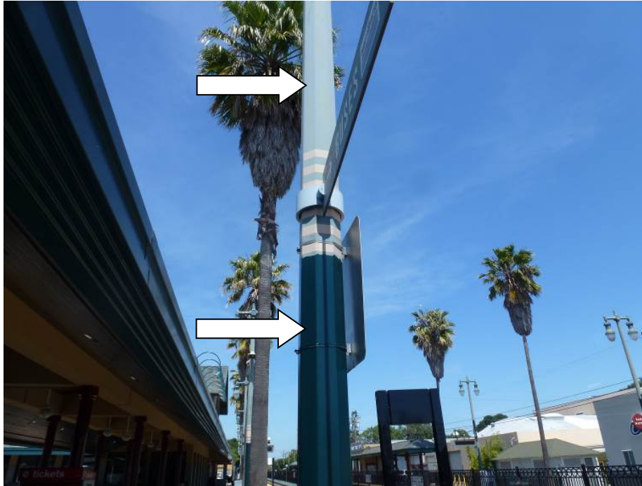
Before & after painted pole along San Mateo platform
