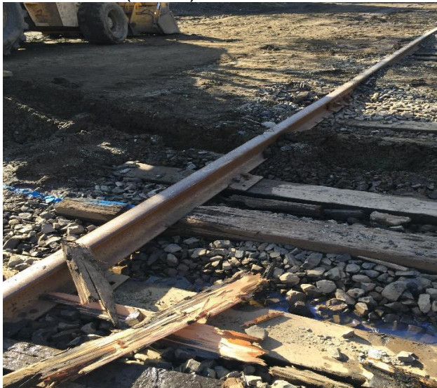
Replacing rotted ties no longer properly supporting the rail in SSFY
