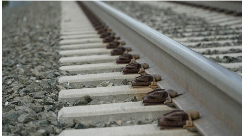
Typical Caltrain track consists of steel rail, concrete ties, and ballast.
