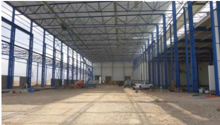
Car Progressive Assembly Area (under construction)
