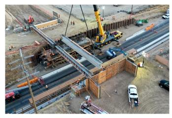
Crews placed the final 12 CP4 pre-cast concrete girders over the State Route 46 underpass in Wasco to create a bridge that will carry high-speed trains. The work is being done to create a bridge that will carry high-speed trains parallel to the BNSF railroad.
