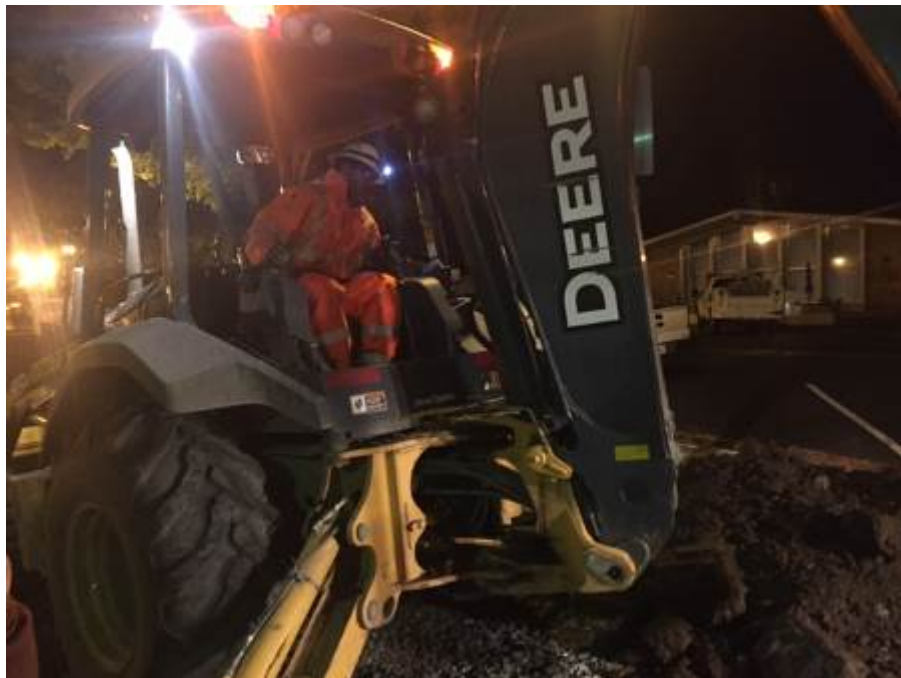
Dug a trench for new Signal conduit and foundation installation
