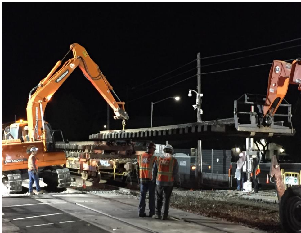
Removed previous rail & ties (track panel)
