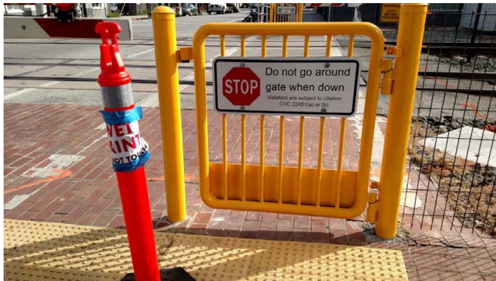
Repainted the swing gates from San Mateo south with "Federal Yellow" for high visibility
