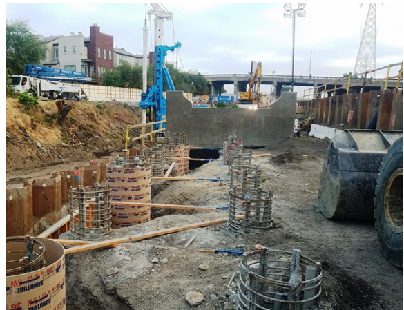
Work stopped during the day as trains passed
