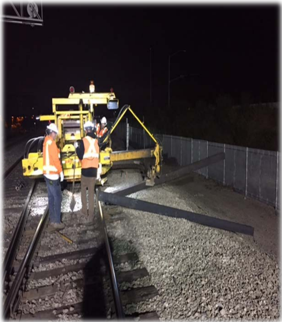
Night work – replacement of ties
