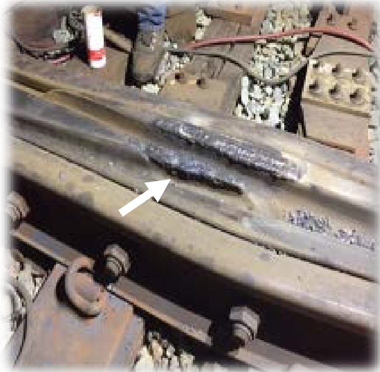
Rebuilt frog point
