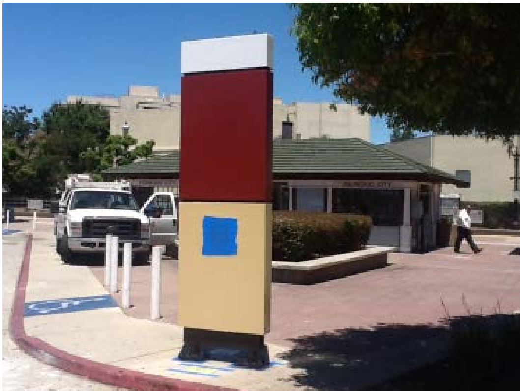
Monument sign work in progress – Redwood City Station
