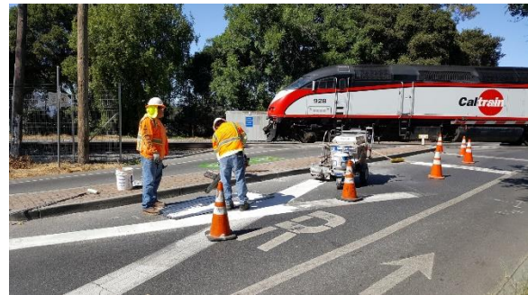
Trains continue without service disruption
