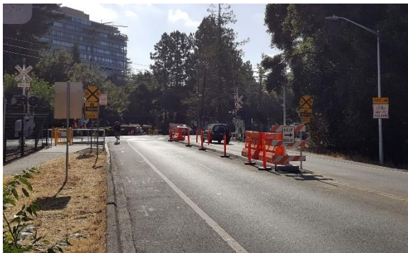
Traffic Control on Palo Alto Avenue Crossing
