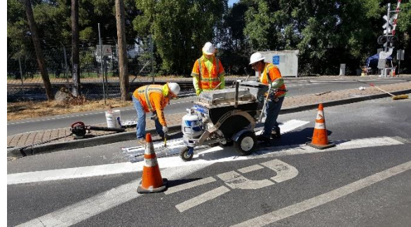
Re-striping with Thermoplastic Paint
