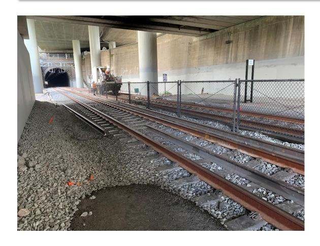
Approximately 5000 Lineal Feet of rail removed and replaced. With no impact to train operations.
