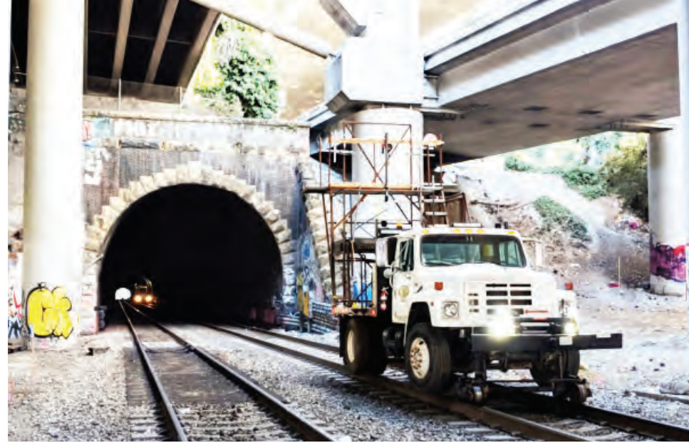
Hi-Rail vehicle for tunnel work in San Francisco
