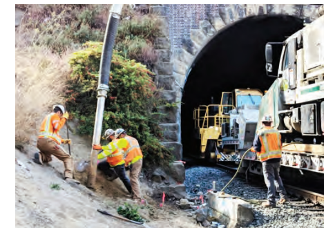
Foundation potholing crew in San Francisco
