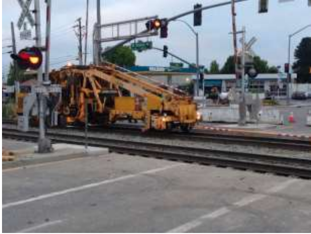
Surfacing and regulating the ballast through the crossing
