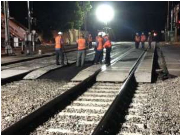
Repaving the grade crossing with asphalt
