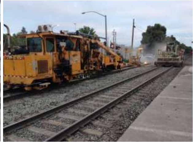
Surfacing and regulating the ballast through the crossing
