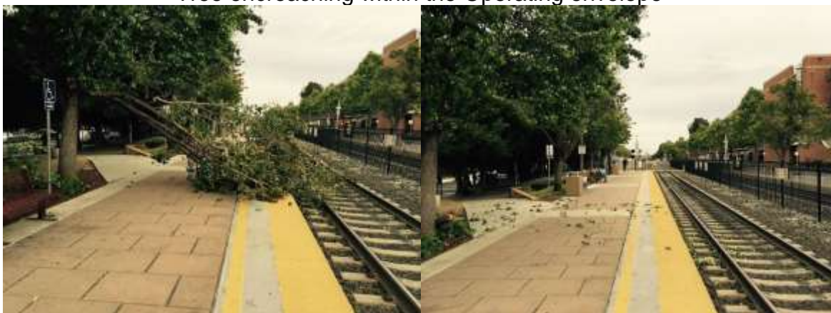
Branches removed and site lines restored
