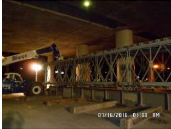
Temporary Utility Support Erection
