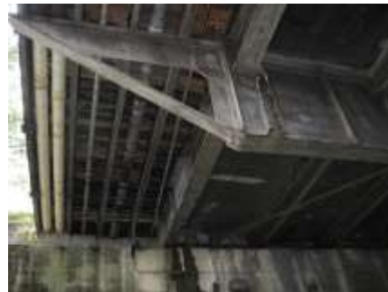
Utility Lines Supported on Existing Structure
