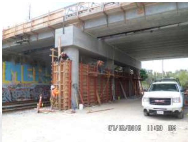
Limits Contractor's Operations
