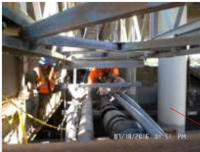
Transfer of Existing Utilities to Temporary Utility Support
