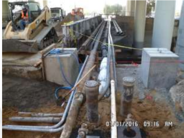
Design modifications made to properly connect to existing utilities
