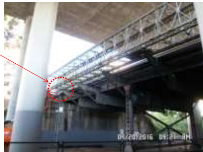
Temporary Utility Support in Place
