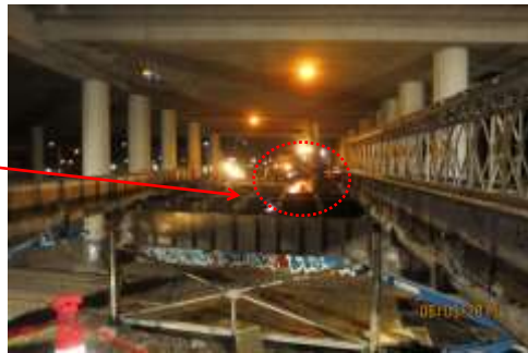
Modified removal method resulted in longer demolition duration
