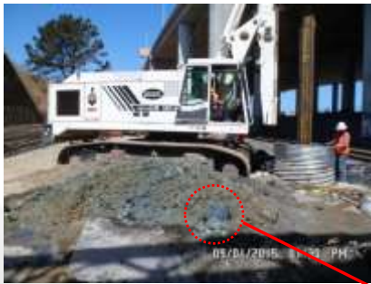
Serpentine with Elevated Levels of Naturally Occurring Asbestos
