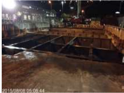
Longer duration to remove concrete deck
