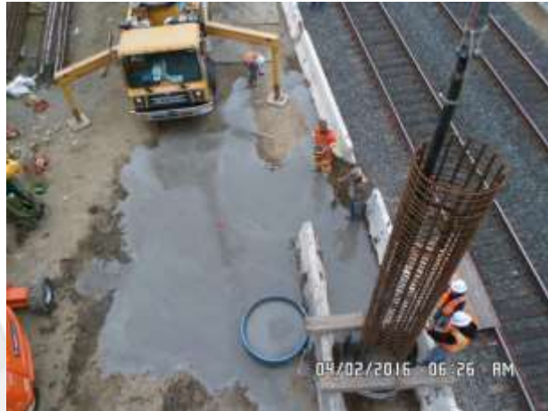
Drilled Pile Installation
