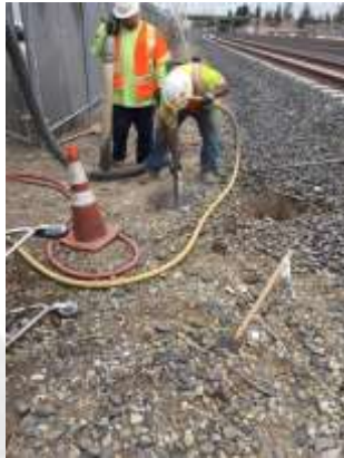
Potholing – to identify utilities
