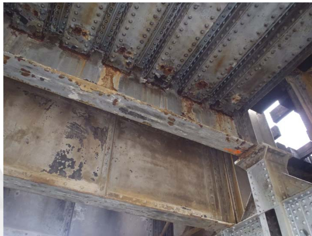
Floor beam corrosion and section loss
