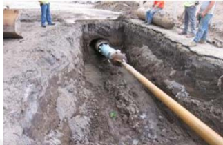
Boring (required at many crossings, within the Caltrain right of way)
