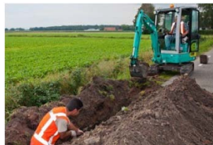
Trench (with mini excavator or by hand, within the Caltrain right of way)
