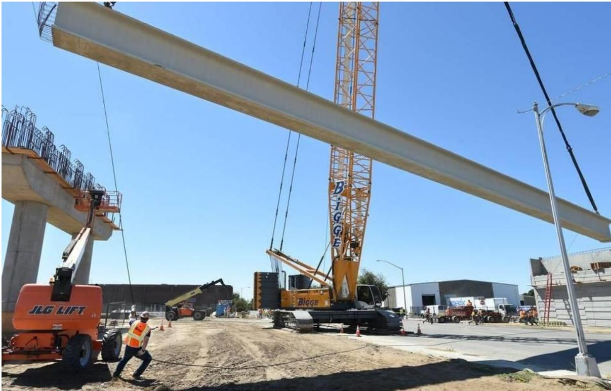
A crane lowers 146-foot, concrete and steel girder, weighing 166,000 pounds, into place as the Tuolumne Street bridge in downtown Fresno was replaced to facilitate the high-speed rail station being built in the city. It will include a stop in Merced when complete. **JOHN WALKER**
