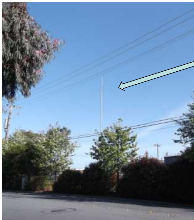
Example 80' pole already on right of way
