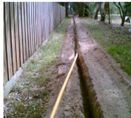
Conduit placed in trench (~42" deep x 9.5" wide, within the Caltrain right of way)
