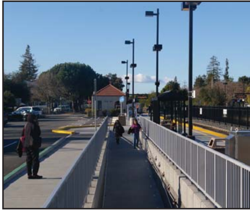
The California Avenue station features a new pedestrian underpass.
