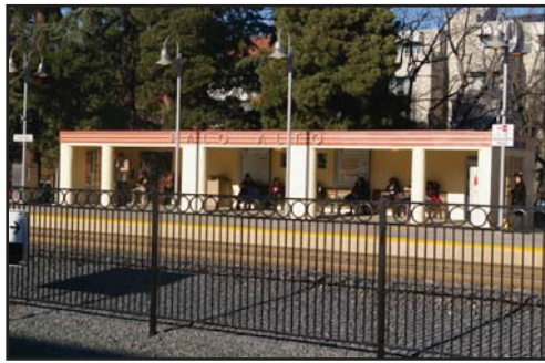
The Palo Alto station received new boarding platforms as part of the multi-million dollar improvement project.
