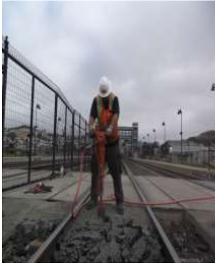
Asphalt and Concrete Panels removed
