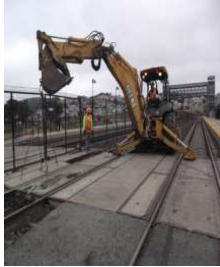
Asphalt and Concrete Panels removed
