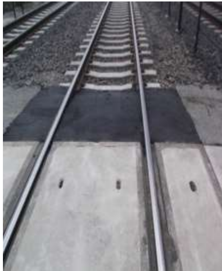
Surfaced track, and installed concrete panels and new asphalt
