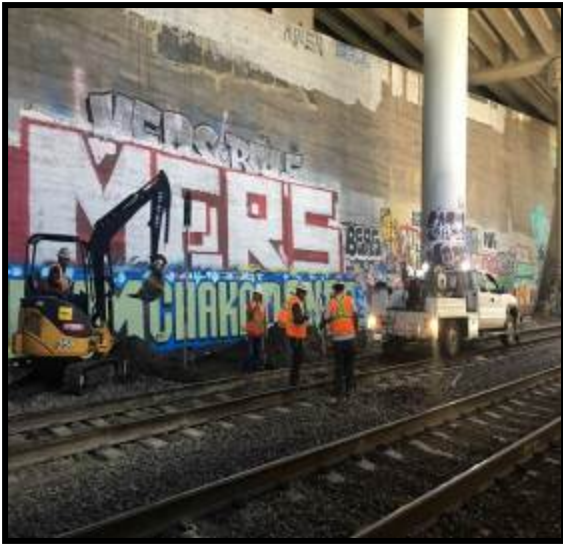
Removed & replaced the fouled ballast and restored the drainage ditch to let the water flow
