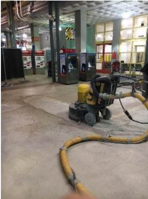
Removal of the existing flooring; had multiple layers built up over the years
