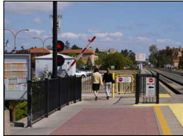
Pedestrian gates at station
