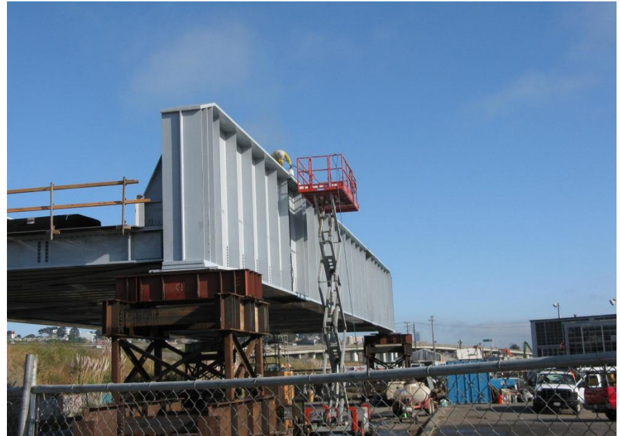
Jerrold Street Bridge - 2011
