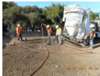
Test pile installation in preparation for foundation installations
