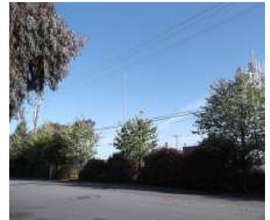
Base Station in Right-of-Way
